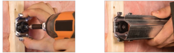
Figure 7: Installation of Pliteq GenieClip RST
