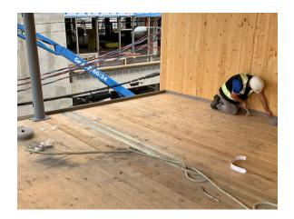
**Step 2:** Begin to roll out GenieMat® FF layer(s) and stagger the seams in a brick like pattern.
