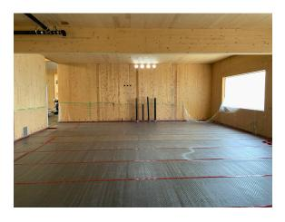
**Step 4:** Pour concrete directly onto the GenieMat® FF system.
