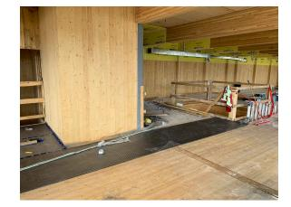
**Step 3:** Using GenieTape, tape all the seams to seal the GenieMat\* FF system when a concrete topping is to be applied.
