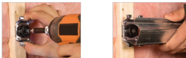
Figure 7: Installation of Pliteq GenieClip RST
